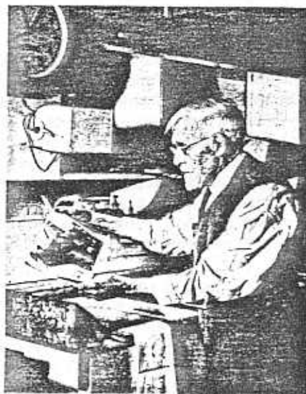
At the age of 97, William H. Jackson, a father of photography, is shown trying his hand in the darkroom of the Department of the Interior. He was official photographer for building of first transcontinental railroad.
